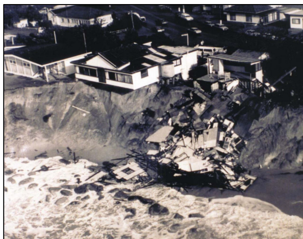
Figure 3: House collapse at Wamberal-Terrigal beach 1978
