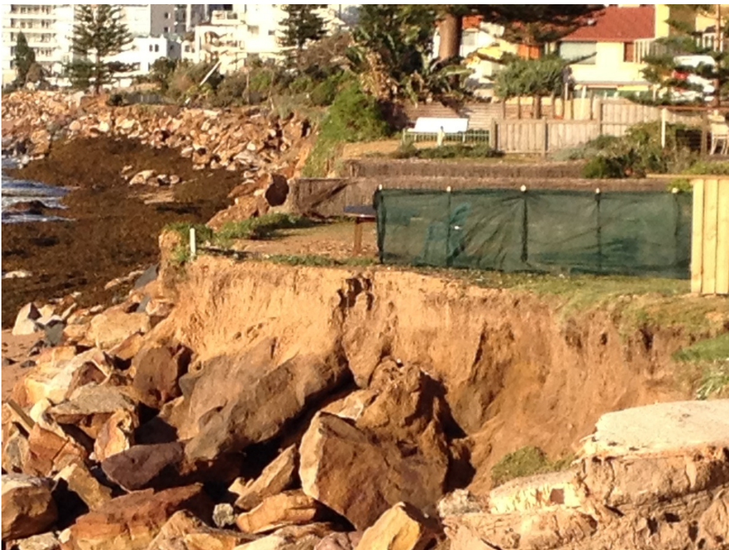
Figure 6: Exposed informal works at Collaroy-Narrabeen Beach
