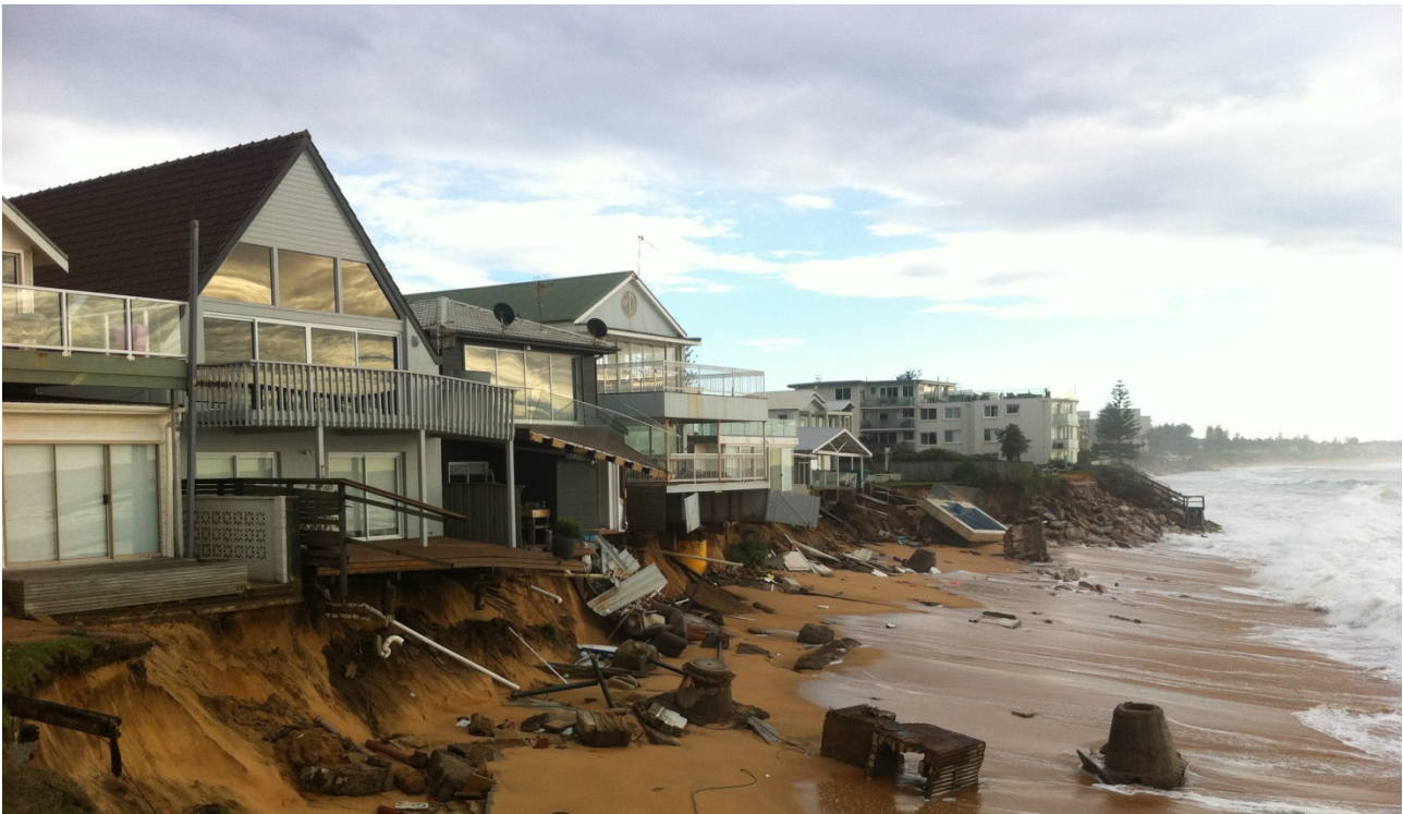
Figure 9: Erosion impacts at Collaroy-Narrabeen June 2016
